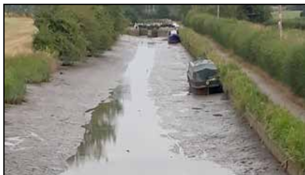
A stretch of the Kennet and Avon canal was accidentally drained this week
