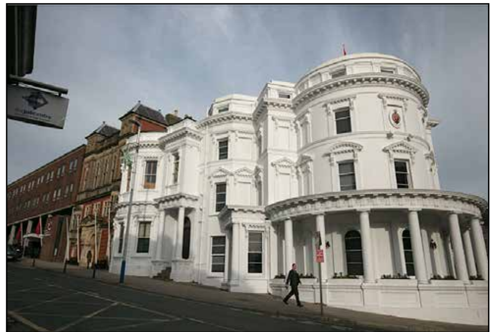
The Tynwald Building, which houses the Manx parliament on the Isle of Man
